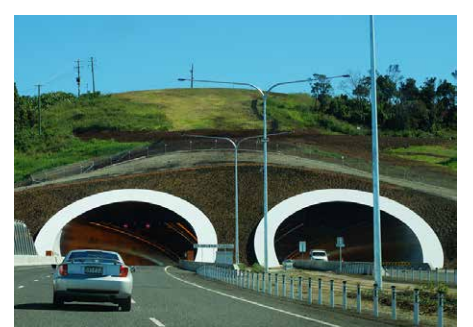
St Helena tunnel, NSW. Example of the intended road tunnel entrance (Skyscraper City 2015).
